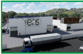
Containerized Power House
